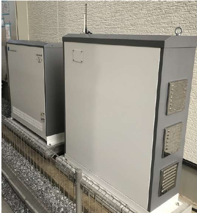
DGR = Digital Grid Router
